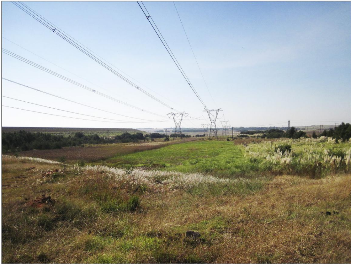
Figure 7: The two incoming lines from the north-east cross a manmade wetland between the Duvha perimeter to the right and a slimes dam visible to the left. See footprint in Figure 1.
