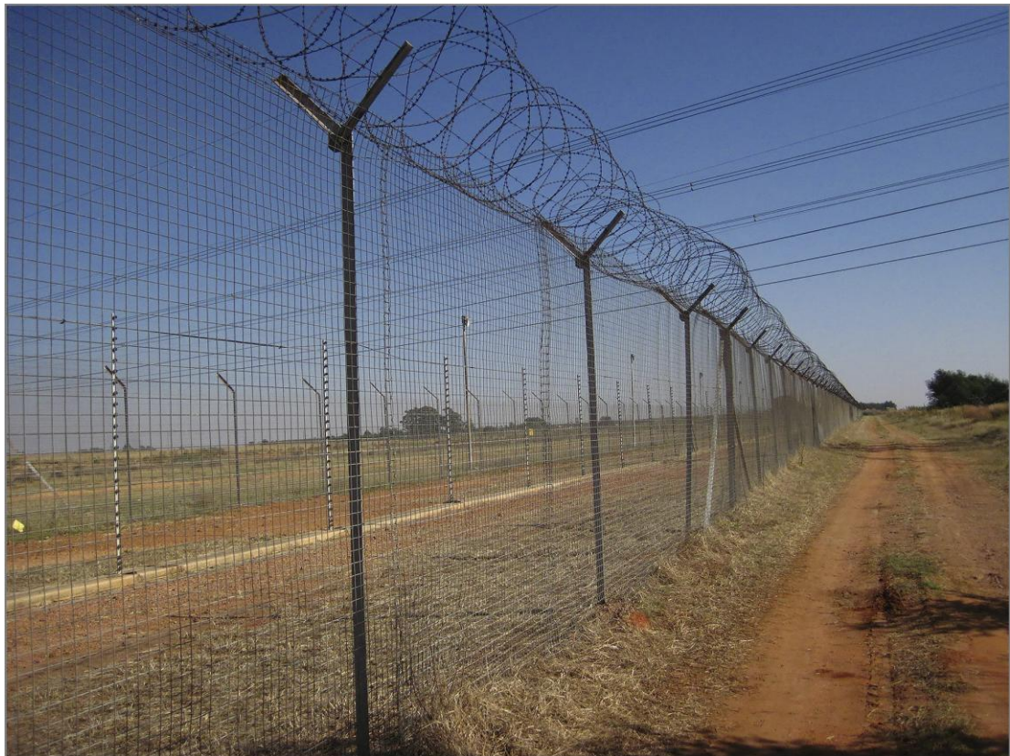
Figure 6: The entire compound of the Duvha Power Station is secured by a double mesh fence with barbed wire loops atop the outer, and an electrical fence in-between.
