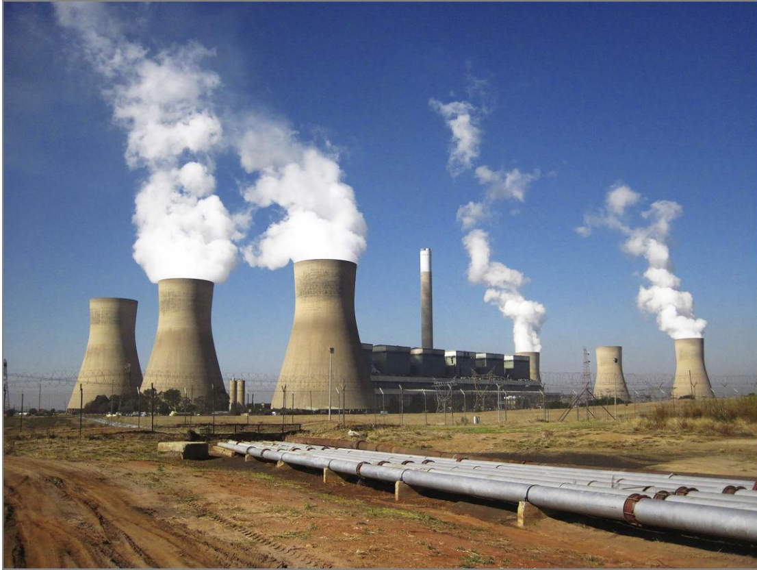
Figure 5: A south-easterly view of the Duvha Power Station. The bypass construction will be within the secured compound of the station.
